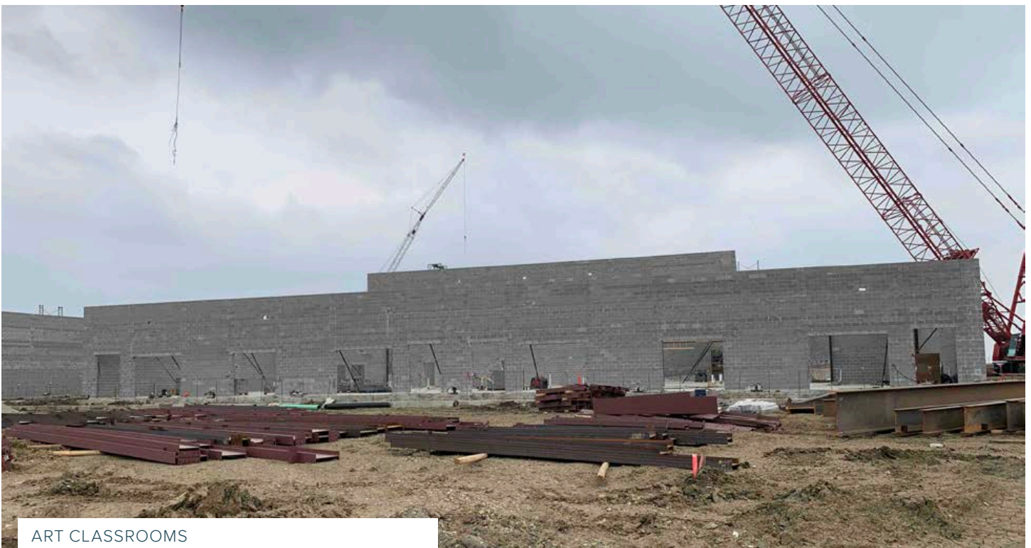
EXTERIOR SHEATHING (WEST ACADEMIC WING)
